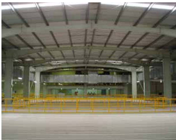
NON-COMPOSITE DESIGN WITH STEEL DECK SUPPORT
