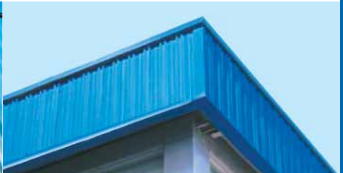
VERTICAL FASCIA WITH BACK UP PANEL AND VALLEY GUTTER
