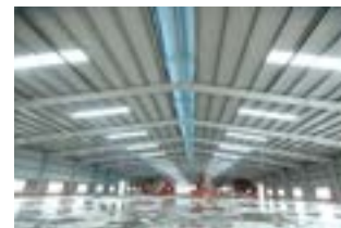
Translucent Panel (Skylight)
