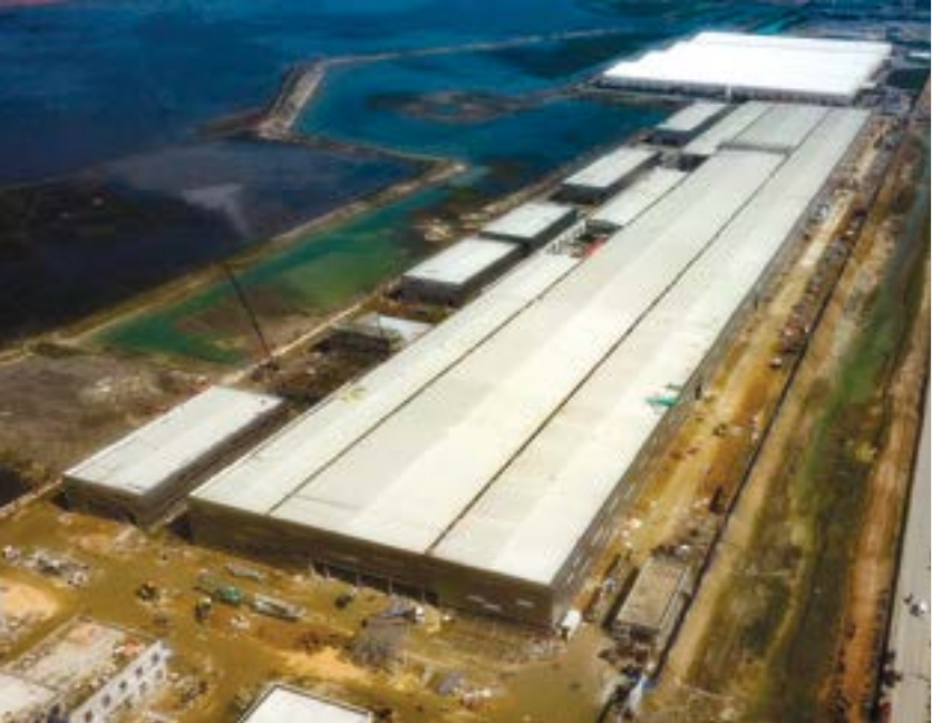
ELECTRIC CAR BATTERY PLANT
