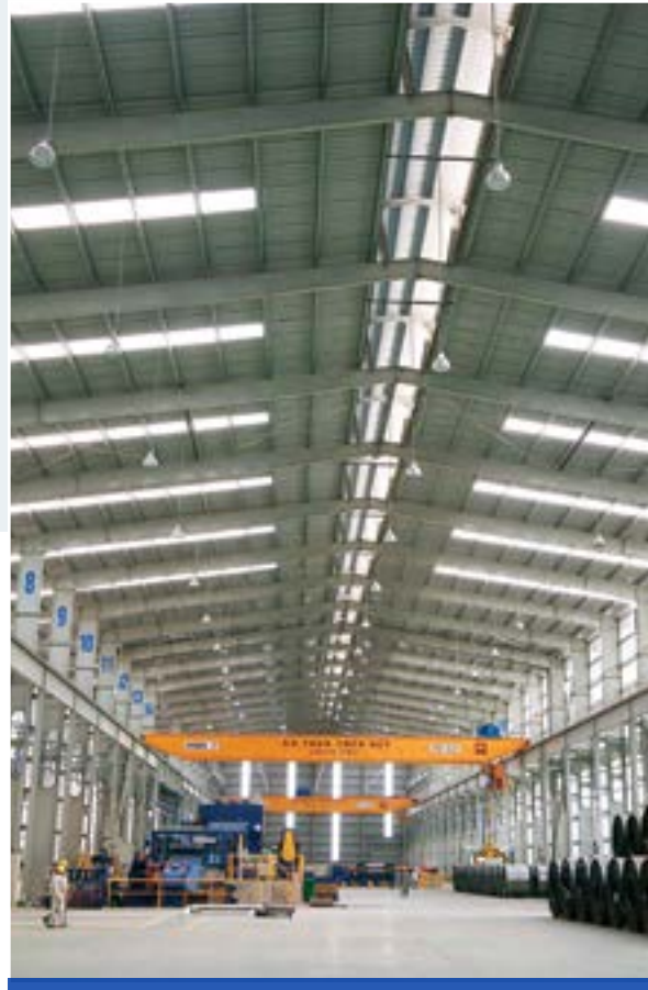
Pre-engineered steel buildings
