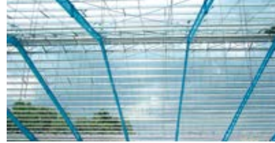
CABLE BRACING
