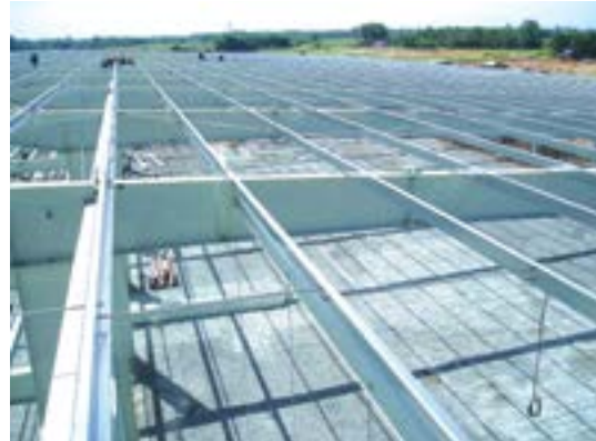
SECONDARY MEMBERS (Minium Yield Strength is 34.0 kN/cm 2 )
