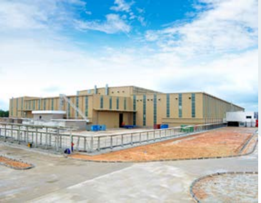
FACTORY IN BATAM ISLAND, INDONESIA
