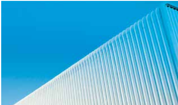
CURVED EAVE WITHOUT PROJECTION (WITH VALLEY GUTTER)
