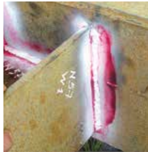
Liquid Penetrant Testing
