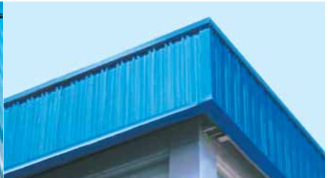
VERTICAL FASCIA WITH BACK UP PANEL AND VALLEY GUTTER
